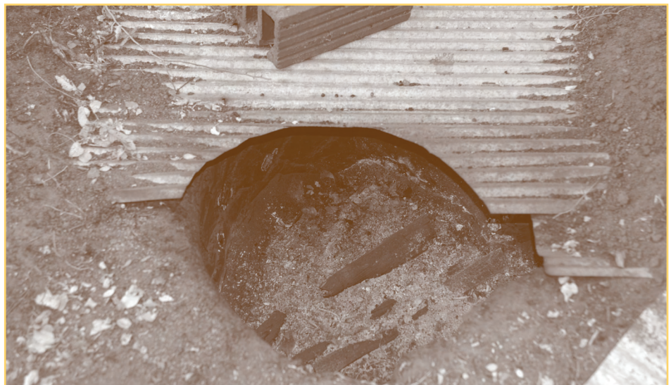
A tunnel, 3 feet out the back of the smoker, is dug out about 18-inches deep. The tunnel is covered with metal and filled over with dirt for insulation. The pit at the end of the tunnel is about the same depth and about 2 feet in diameter. Two pieces of metal cover the pit and make it easy to control the heat.
